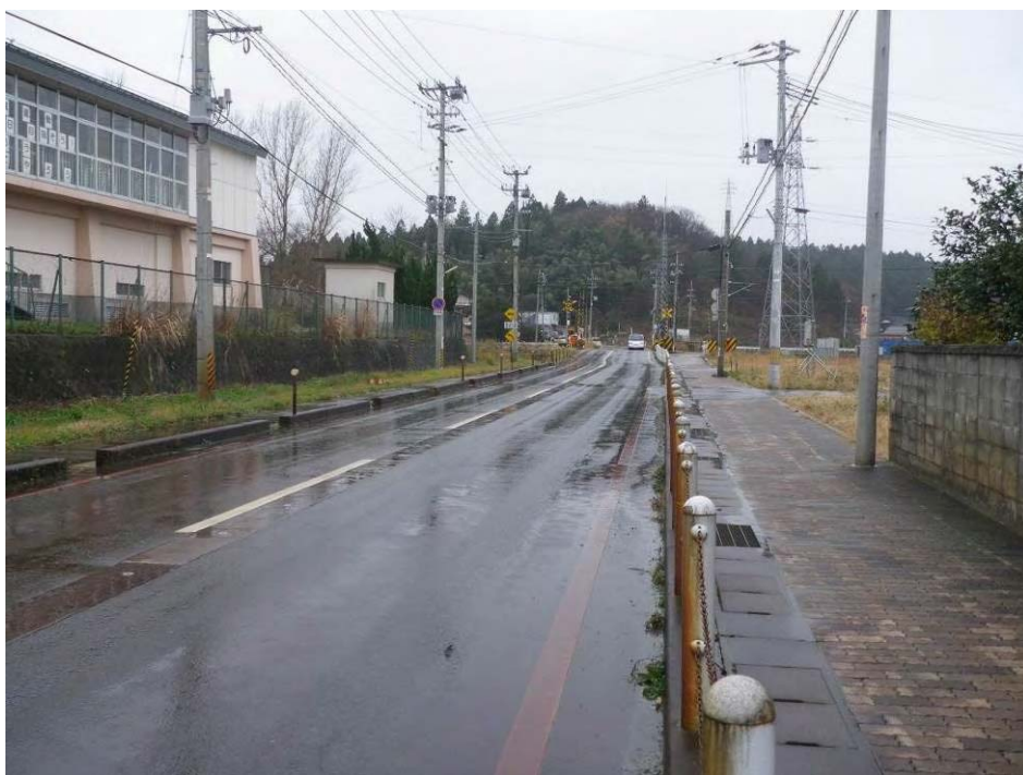
[ (一)岩船港線_岩船街道踏切付近]
