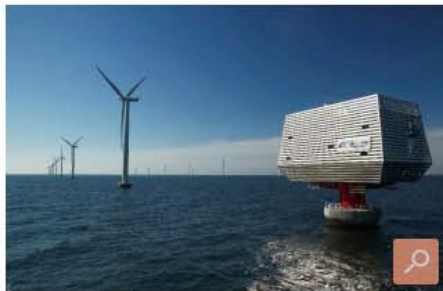
Nysted offshore wind farm (Photo: DONG Energy)
