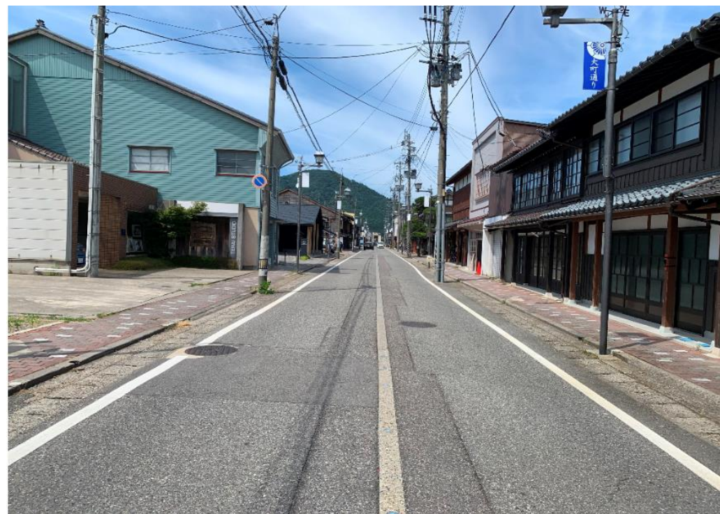
(修理・修景後)
