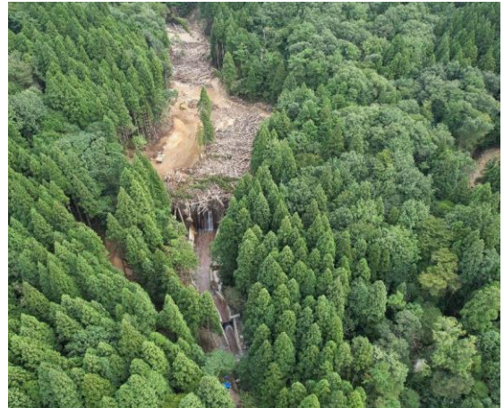
▲小岩内大沢砂防堰堤
